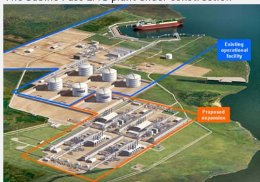
The Sabine Pass LNG plant under construction
