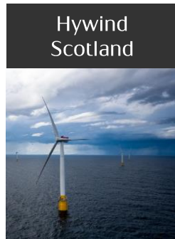
In operation Offshore floating wind
